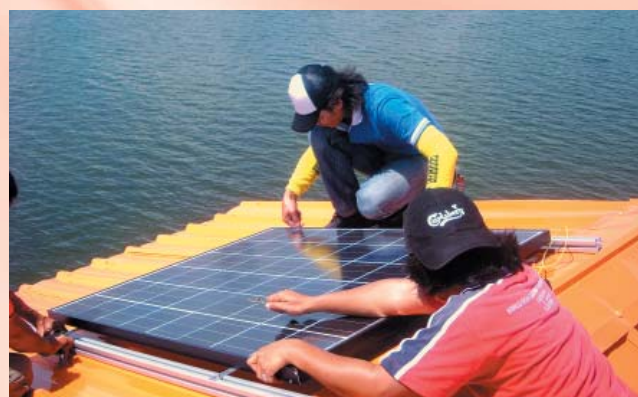
Installation of Solar Light System
